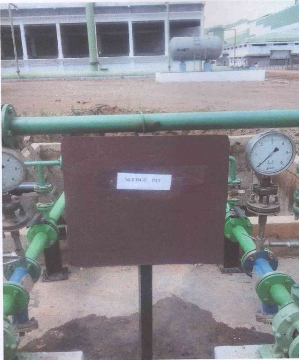
Photo of Sludge Pit.
